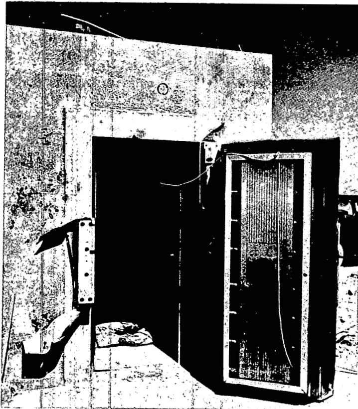
Fig. 8—Front face of vault, door open, postshot.
